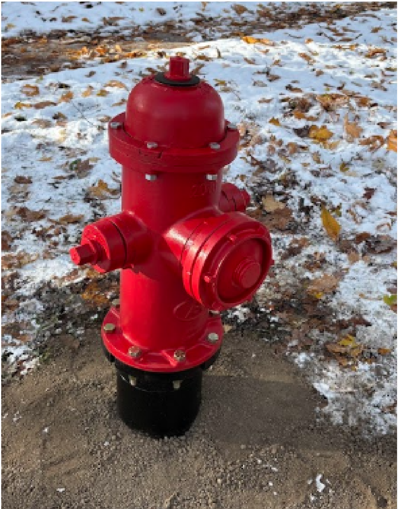
Recent fire hydrant improvement.
